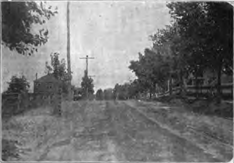
Sayreville road, Middlesex Co., after improvement.
